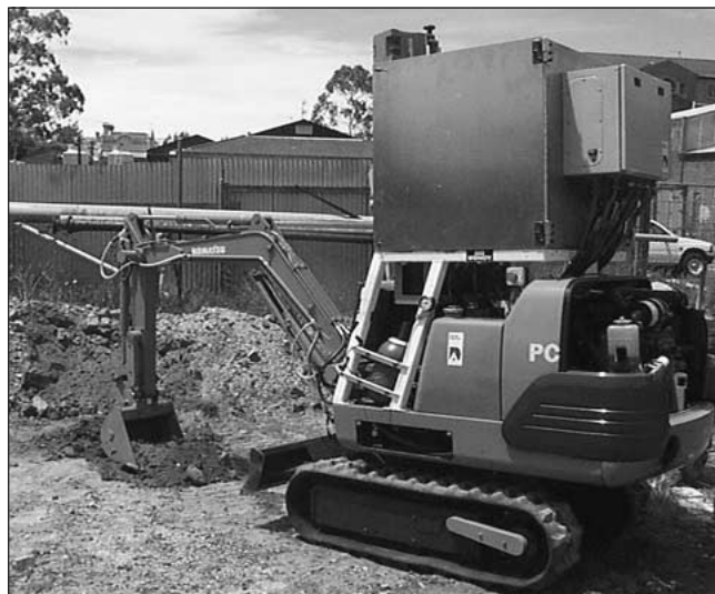
Figure 1. The robotic excavator in a trench-forming task.
