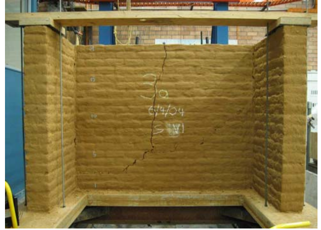
Figure 9. Internal view of wall unit showing stair-step and vertical cracking.
